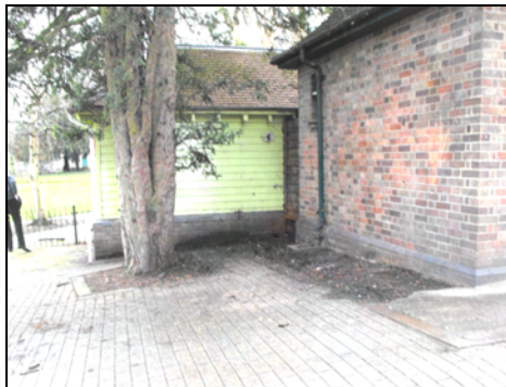
Photo 2.29: Possible location in front of building
